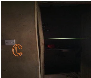
Plate 3: Warping in door post
