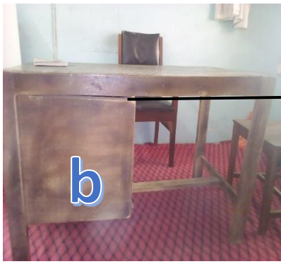
Plate 2: Warping in table-drawer compartment
