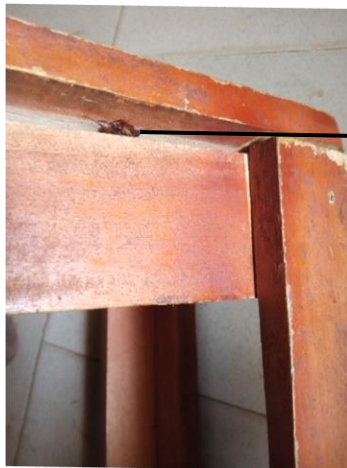
Plate 8: Loosened joints in stool members
