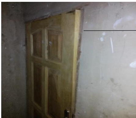
Plate 1: Warping in door leave
